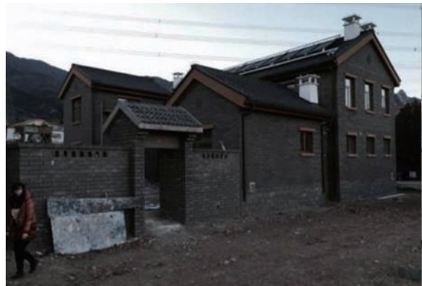
Appearance of 150m 2 house
