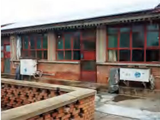
Fig.19 Real Scene of the Outdoor Ground Energy Heat Treasure unit in front of the House
