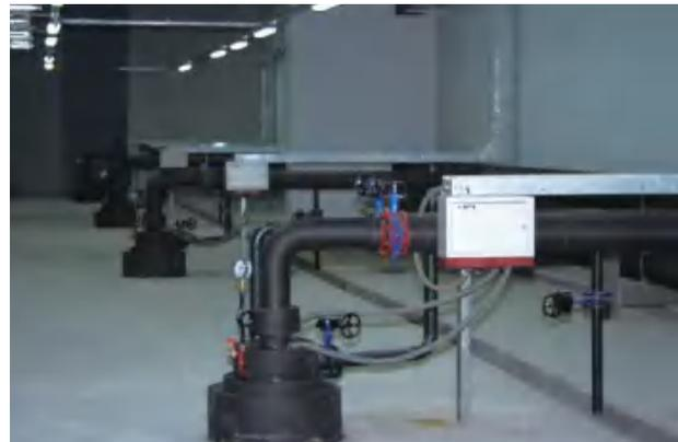
Fig.12 Single Well of Geothermal Energy Collection with Circulation Heat Exchange in the Basement of the National Grand Theatre
