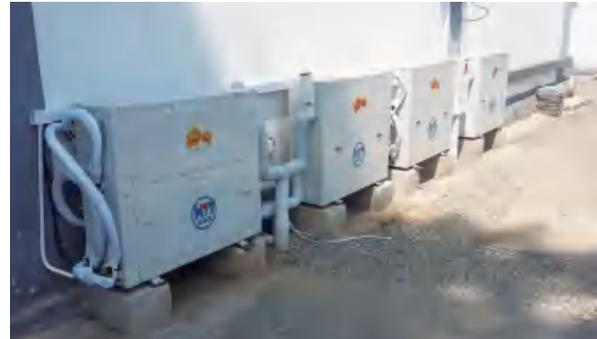
**Fig.17 Real Scene of the Outdoor Ground Energy Heat Treasure unit behind the House**
