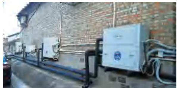
**Fig.16 Real Scene of the Outdoor Ground Energy Heat Treasure unit behind the House**
